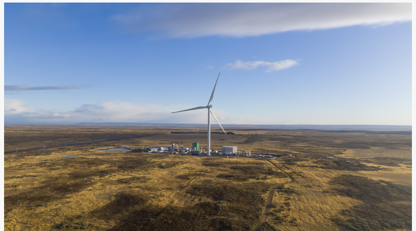
HIF Haru Oni e-Fuels facility in southern Chile
