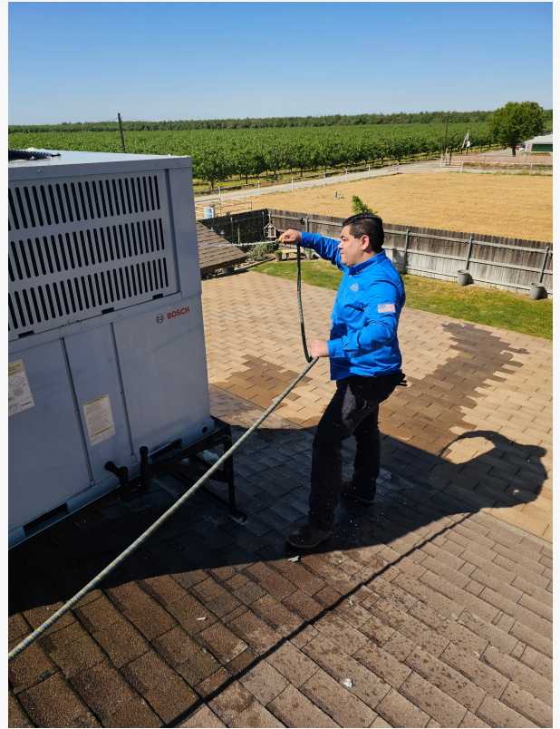
Mechanical Air technician cleaning an HVAC unit to improve efficiency and ensure reliable performance.
