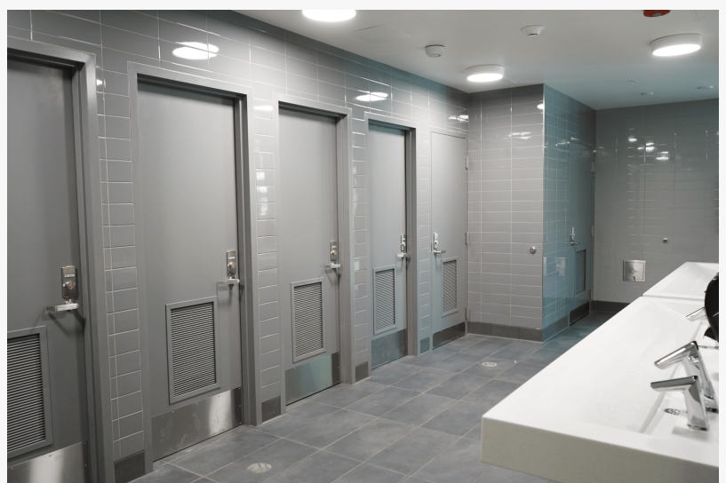
13 Modernized and Upgraded Restrooms
