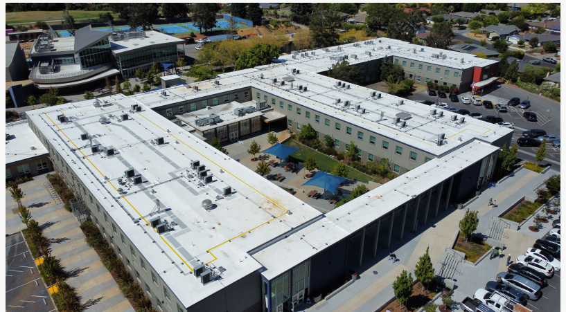
Roof Demolition and Replacement
