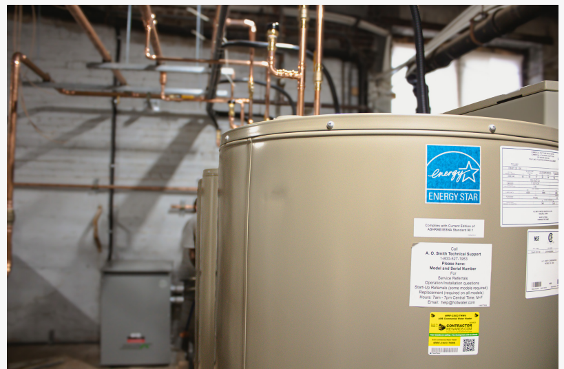
Energy efficiency Shift: replacing appliances and optimizing systems in the residential building of Société immobilière Bélanger in Quebec and Lévis.
