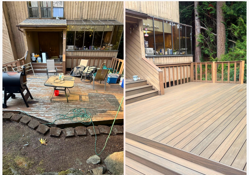
Before & After: Deck Renovation in Everett, WA
