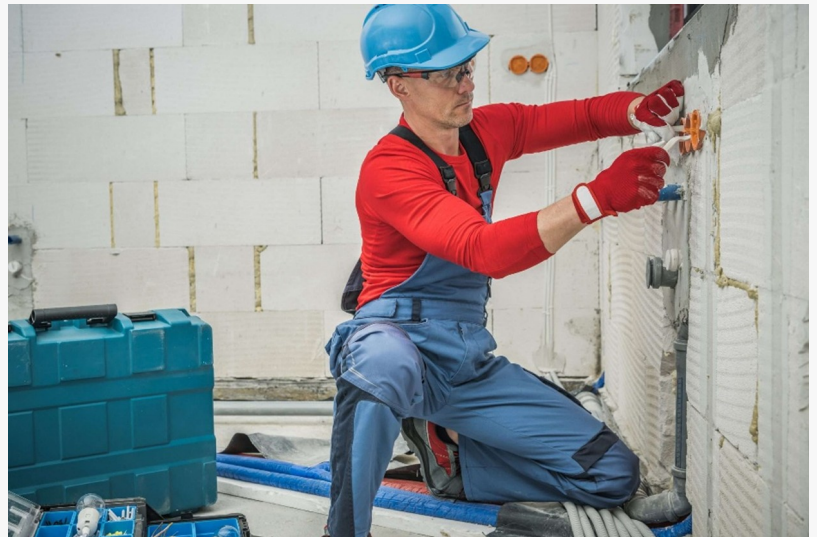
repipe company in San Jose
