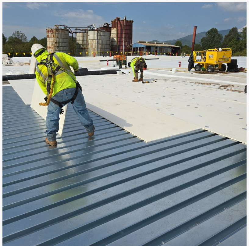
Installing new insulation and metal decking on an industrial roof
