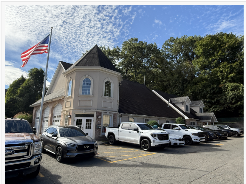
Former Firehouse, N Haledon
