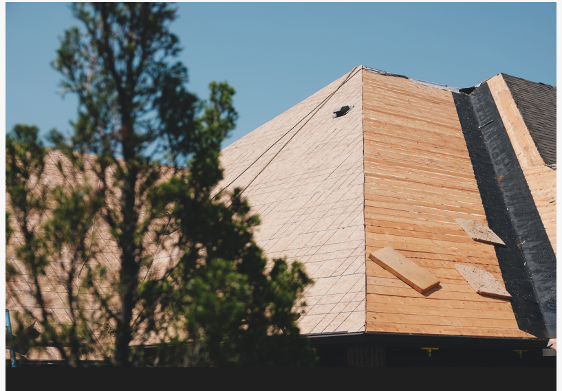
New Roof Installation
