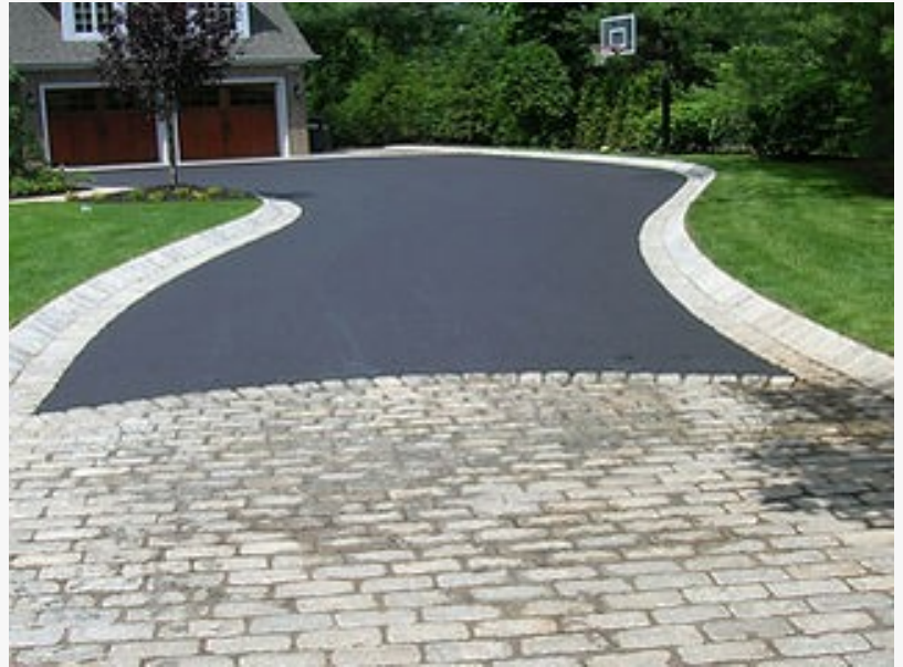
Landscape Construction in Bloomfield, NJ
