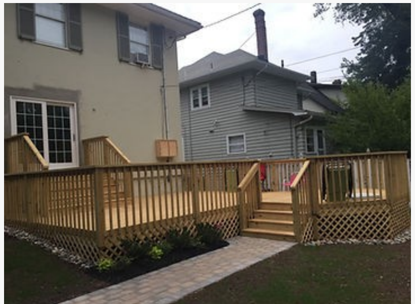
Deck Construction in West Orange, NJ
