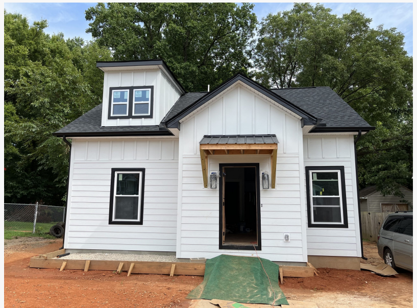
Arctic White James Hardie® siding on a newly built home, installed by Hatch Homes in North Carolina.
