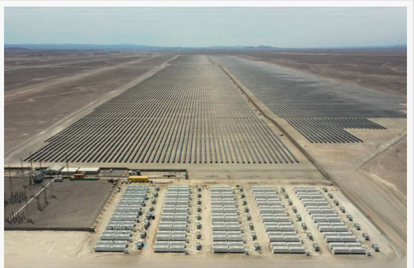
Renewable Energy Project in the Atacama Region Transforms Chile
