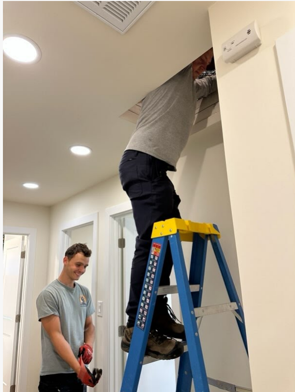
Future Generation Construction getting to work on a home remodeling project for an attic
