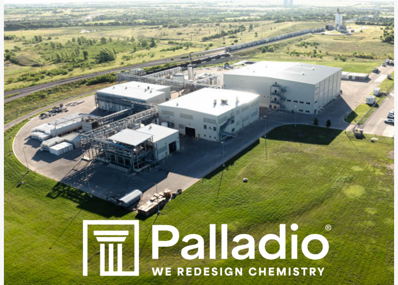
Palladio Industries Industrial Plant in Temple Texas
