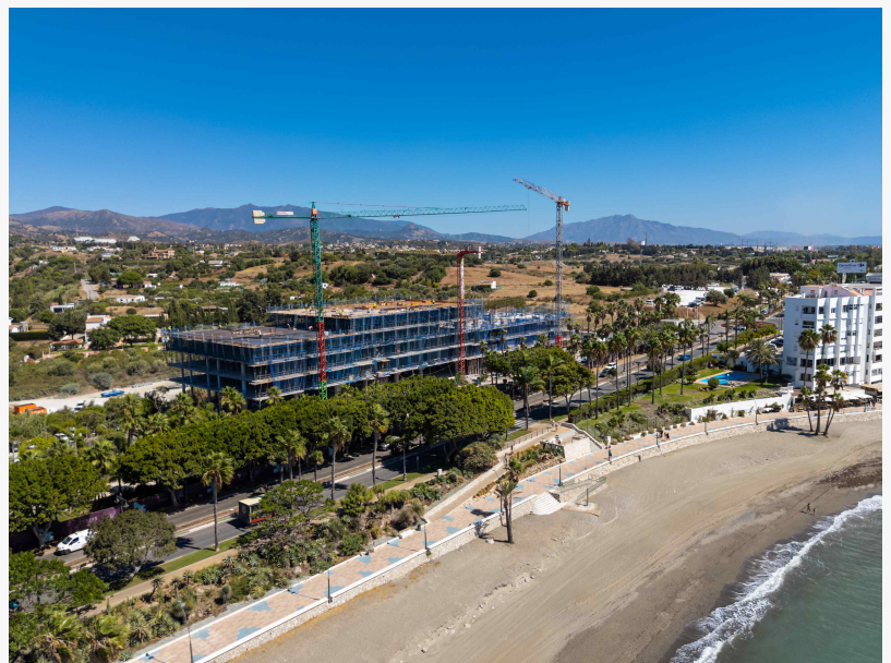
Construction works for Tyrian Residences
