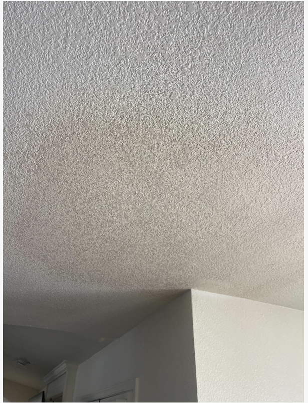
Water damage repair textured and paint-ready
