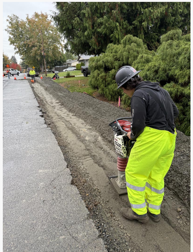
Compaction of Soil being done by In-Depth Excavation
