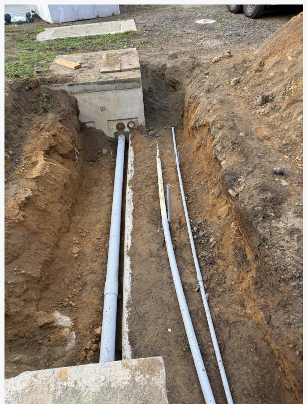
Excavation Job for Utility Trenching with InDepth Excavation
