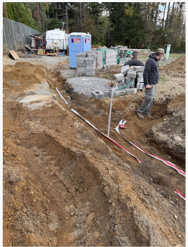
Utility line trenching preparation with In-Depth Excavation
