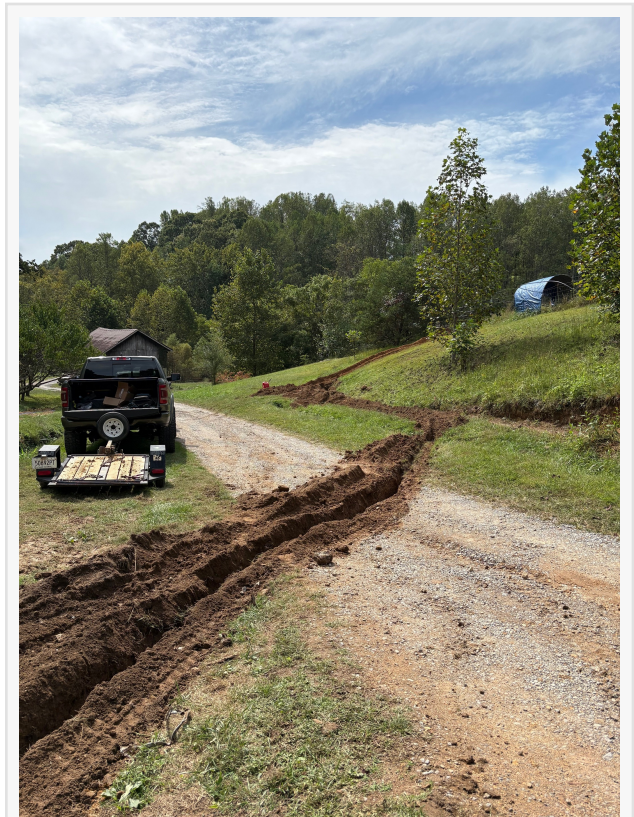
Land Clearing and Excavation work with Jefferson Land Clearing and Excavation
