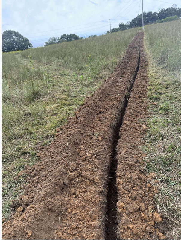
Site preparation for utility lines with Jefferson Land Clearing and Excavation
