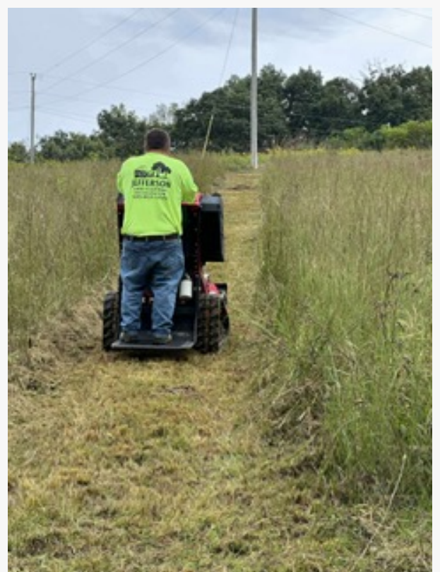
Steven from Jefferson Land Clearing and Excavation trenching for utility lines for site preparation project
