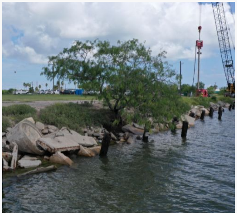
Original Seawall Constructed in 1965
