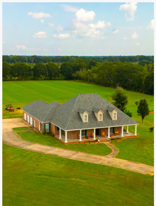
Fortified Roof Lafayette Louisiana
