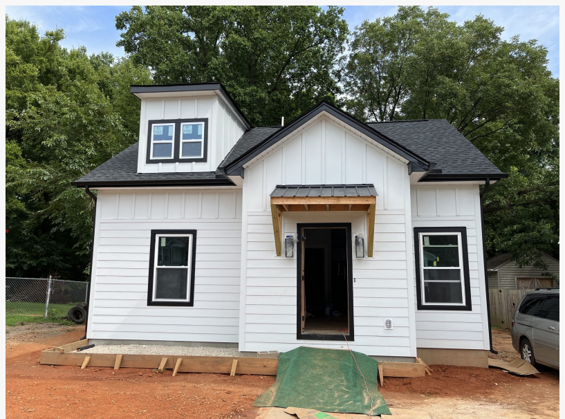
New Construction Featuring White James Hardie Siding
