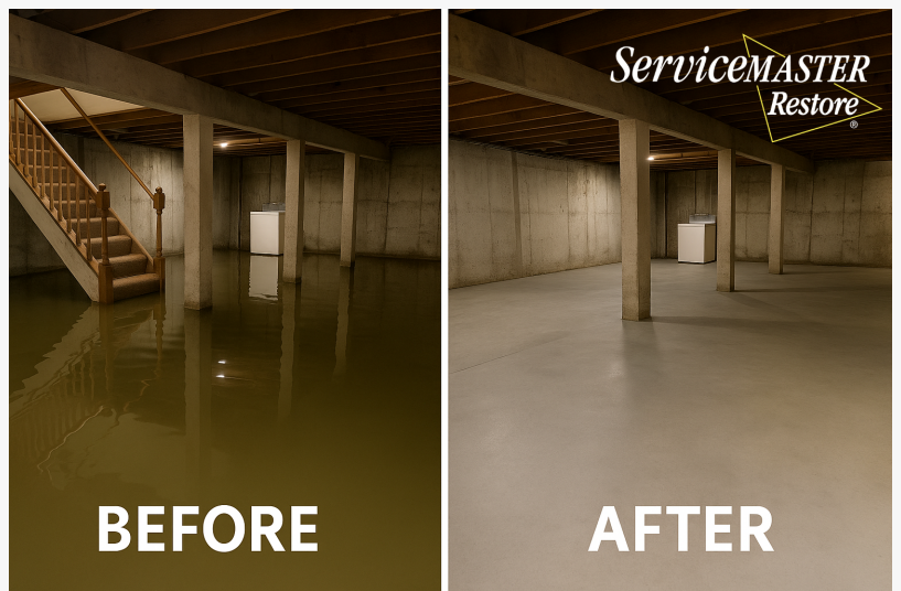
a side-by-side photo of a flooded basement after it has been cleaned and disinfected
