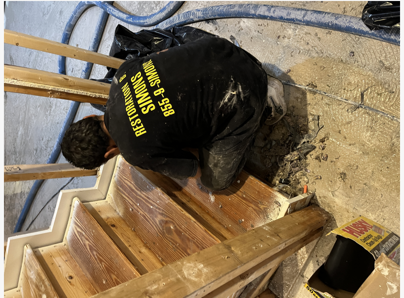
A ServiceMaster Restoration By Simons technician removes wet carpet and debris from a staircase after a water loss in Lake Forest, Illinois.
