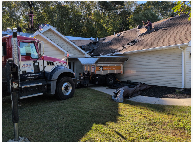
Loading the shingles onto one of the housing units to begin the replacement.
