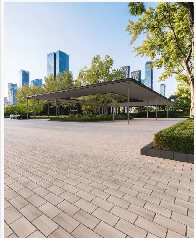
Commercial parking using Techo-Bloc's permeable pavers
