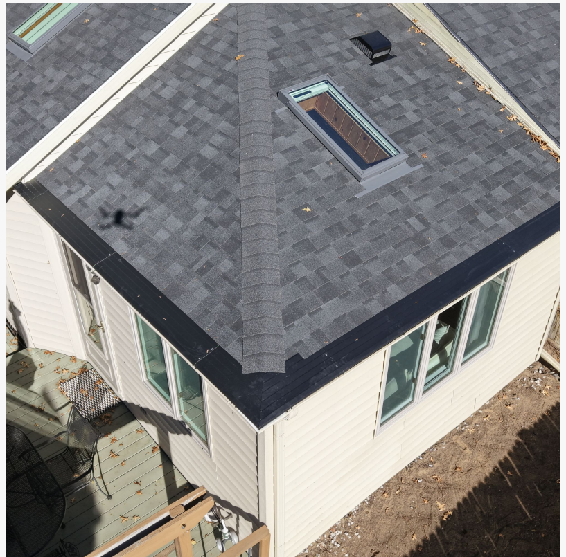
Aerial view of a recently completed asphalt shingle roof with seamless black gutters and a skylight, installed by All Exterior Solutions in Toledo, Ohio.
