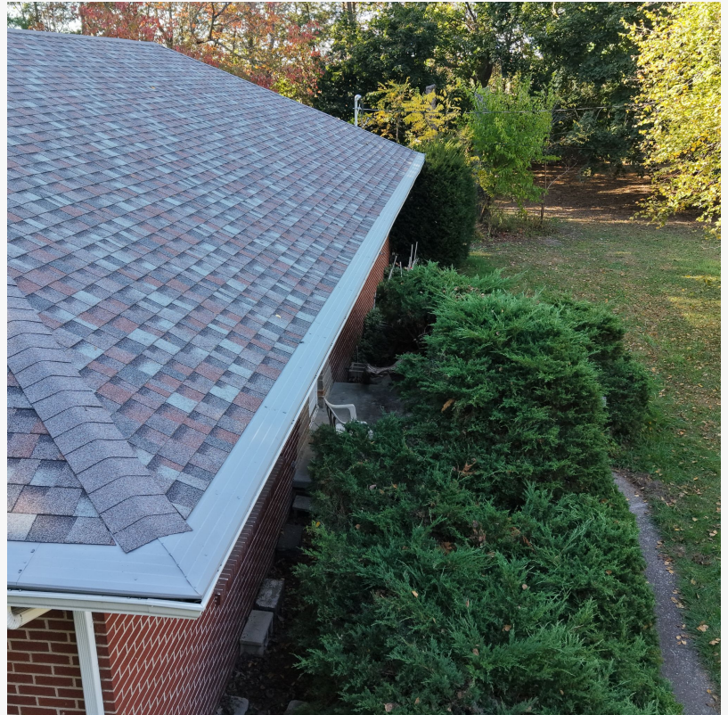
Oblique aerial of a newly installed architectural shingle roof with seamless gutters and gutter guards on a brick residence completed by All Exterior Solutions in Toledo, Ohio.
