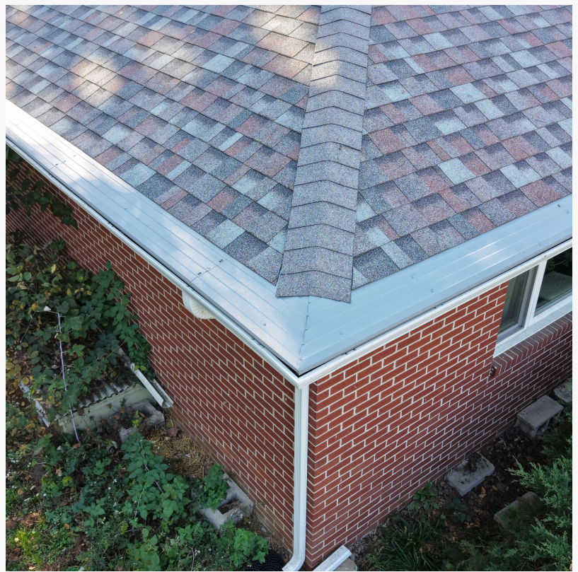
Aerial view of a newly installed architectural shingle roof with seamless white gutters and gutter guards on a brick home in Toledo, completed by All Exterior Solutions.
