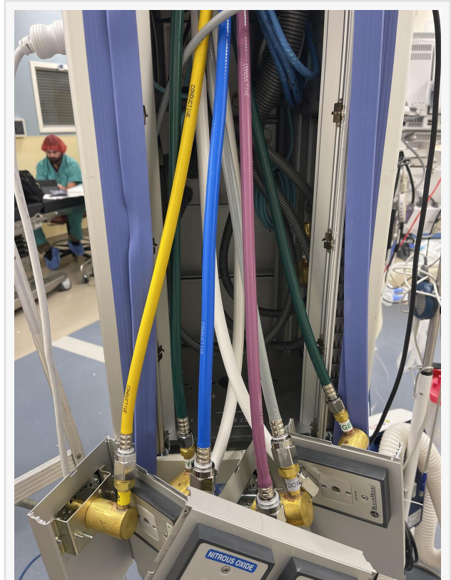
Medical Gas Hose Repair
