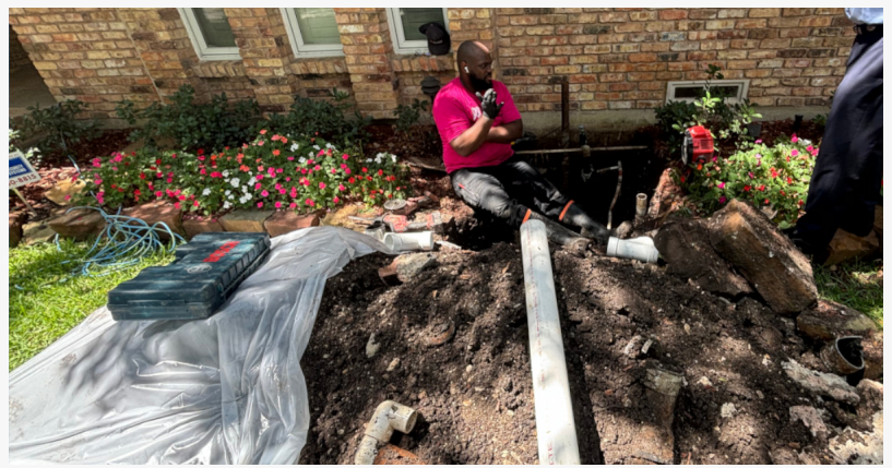
Mother Modern Plumbing replaces cast iron pipe in Fort Worth home.
