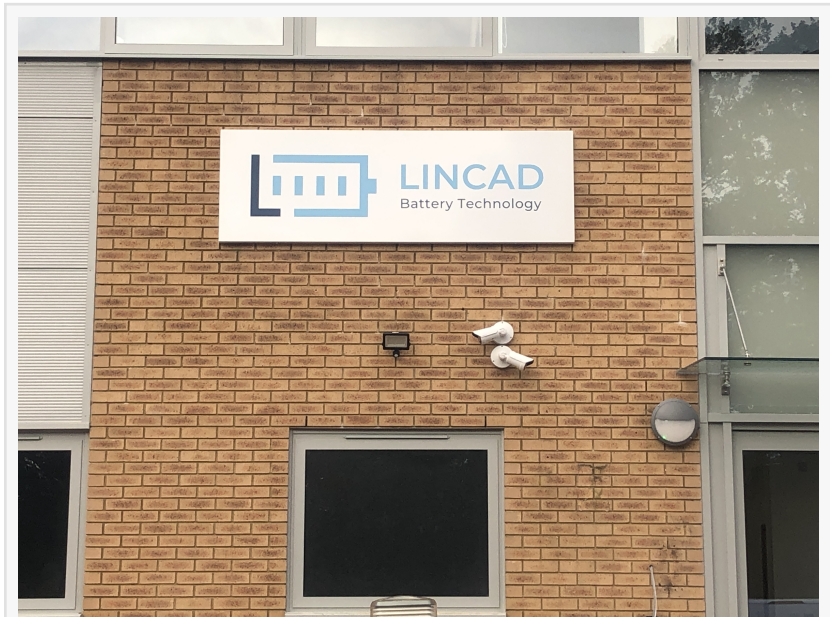
Lincad opens rebuilt State-of-the-Art facility in Ash Vale, marking fresh era of growth
