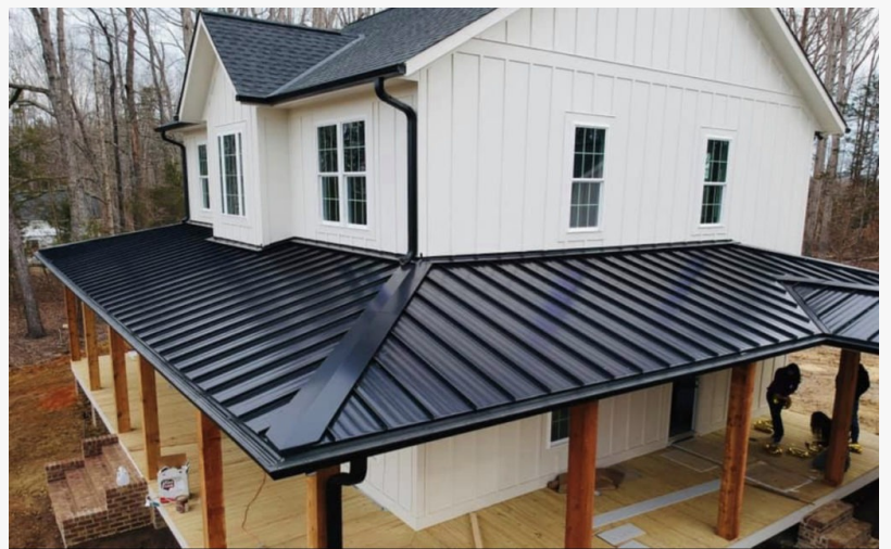
Alt text: well-maintained metal roofing system representing Alpine Roofing's commitment to storm preparedness and roof safety across North Texas
