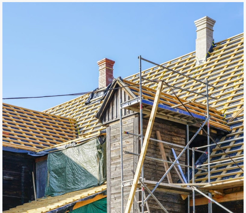
roof replacement in progress
