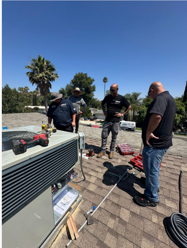
HVAC Contractors Los angeles
