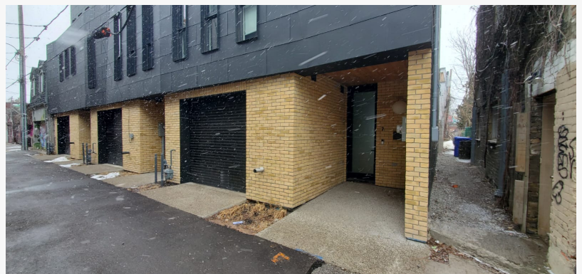
Freshly laid brick wall construction with clean mortar joints in Toronto
