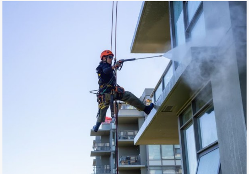
construction pressure washing
