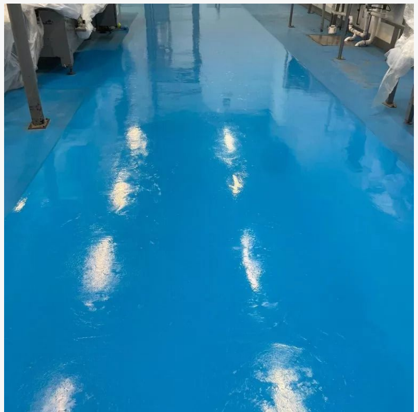
Epoxy Floor Installers
