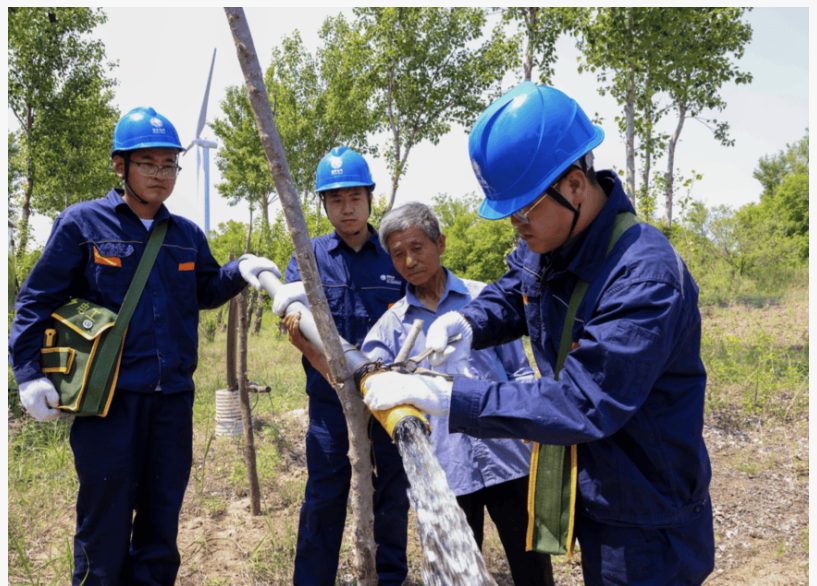
Power company employees conduct on-site line inspections and repairs while assisting local villagers in the forested area.
