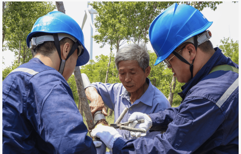
State Grid Fuxin employees work closely with local residents to restore and electrify irrigation systems that support new tree growth.
