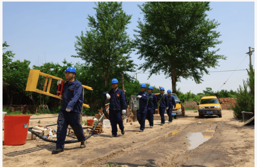
Power supply workers from State Grid Fuxin carry equipment and materials through the reforestation zone to maintain and upgrade rural power lines.
