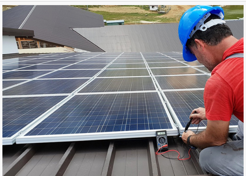
solar panels and roof damage-
