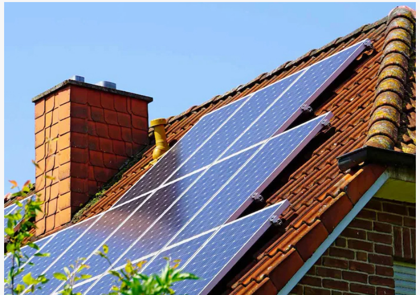
roof shingle solar panels
