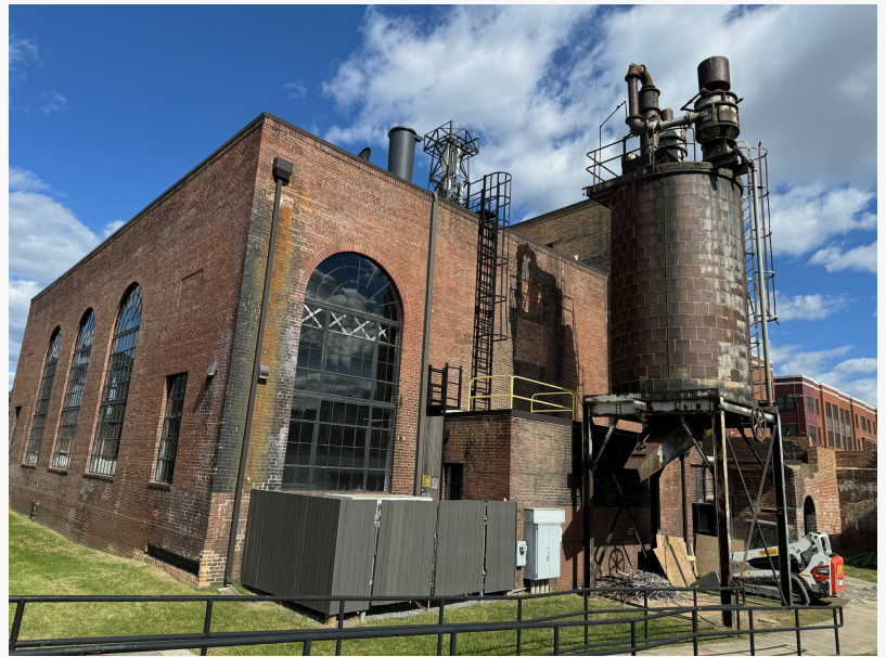
The Power Plant at Liberty
