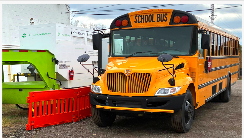
Pontiac EV bus being charged by L-Charge Unit
