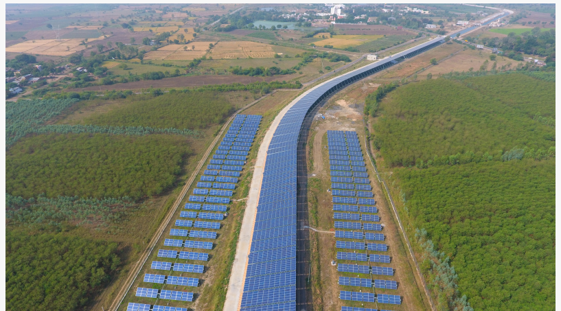
Asia's largest canal-top solar plant — Narmada Canal Top, Gujarat (Capacity: 15 MW)
