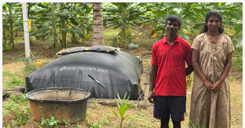
8 cubic meter biogas plant in rural India
