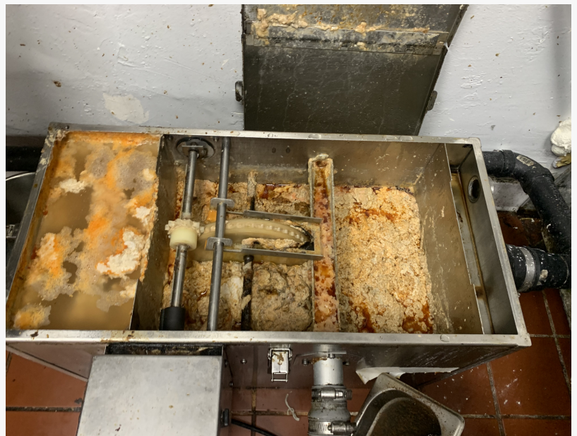
Technicians performing grease trap cleaning, removing fats, oils, and grease to maintain safe wastewater flow.
