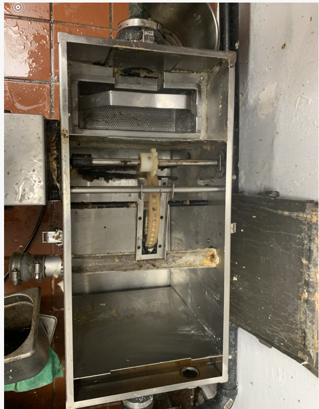
After a successful grease removal service, a clean grease trap in a restaurant of San Diego
