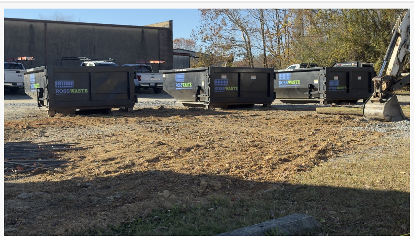
Construction begins at WNC Roofings Fletcher, NC Office
