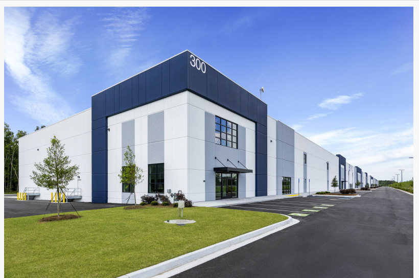
Central Port Logistics Center in Savannah, GA
