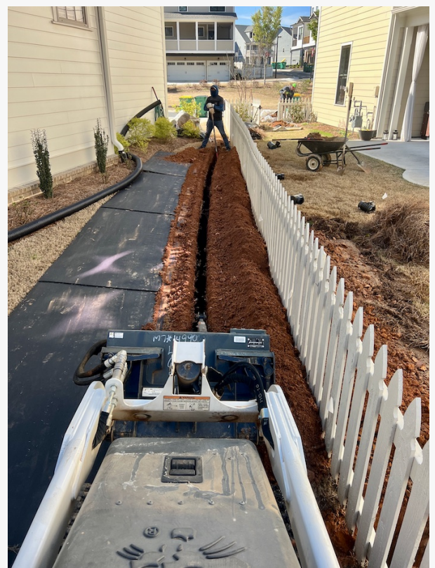
Professional Landscape Drainage Solution Installation
