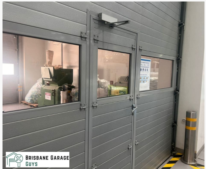
Professional Garage Door Repair in Brisbane
