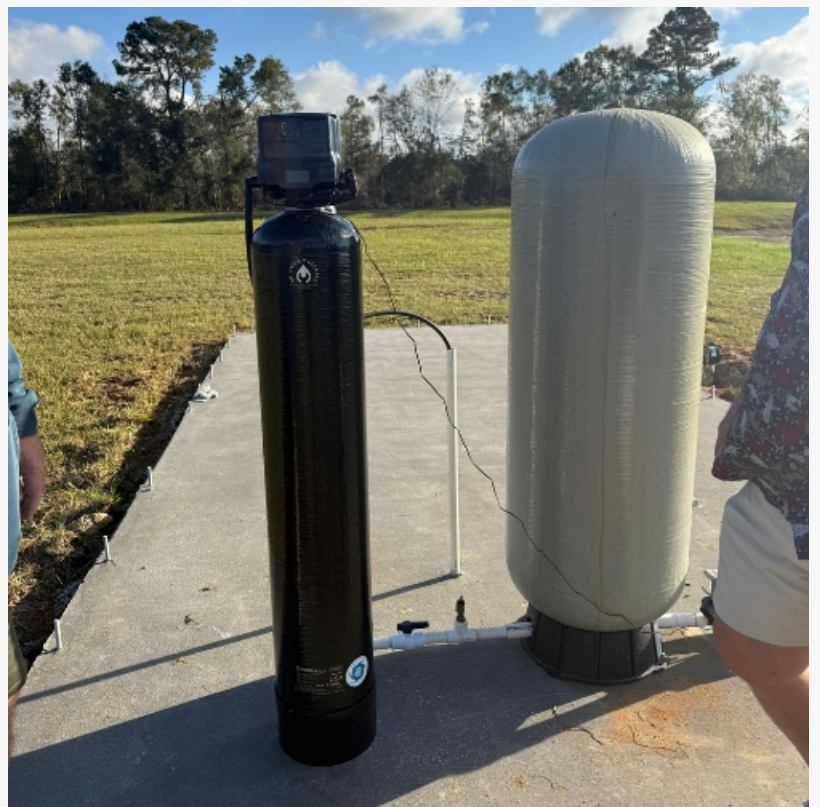
A newly installed outdoor filtration unit and pressure tank by SK Water Wells, built to deliver clean, reliable water for Mississippi homes
