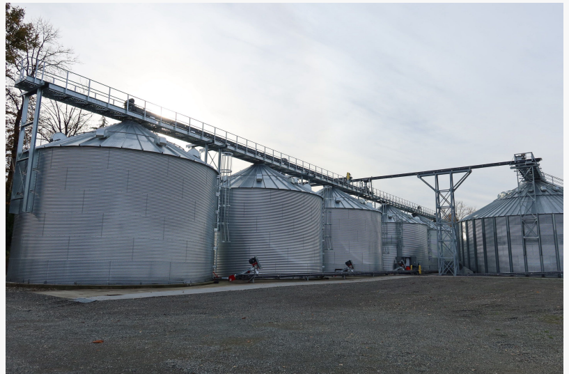
Granary Expansion Project Port of Skagit
