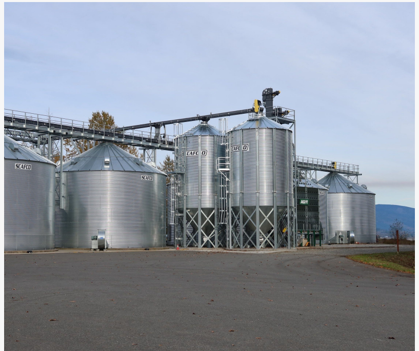
Granary Expansion Project Port of Skagit 2
