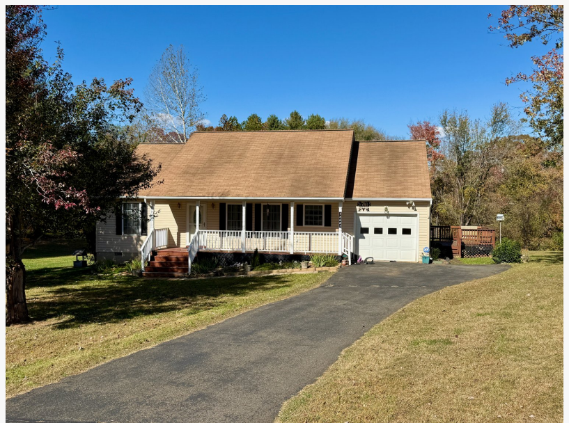
18607 Springs Rd., Jeffersonton, VA (Culpeper County)
