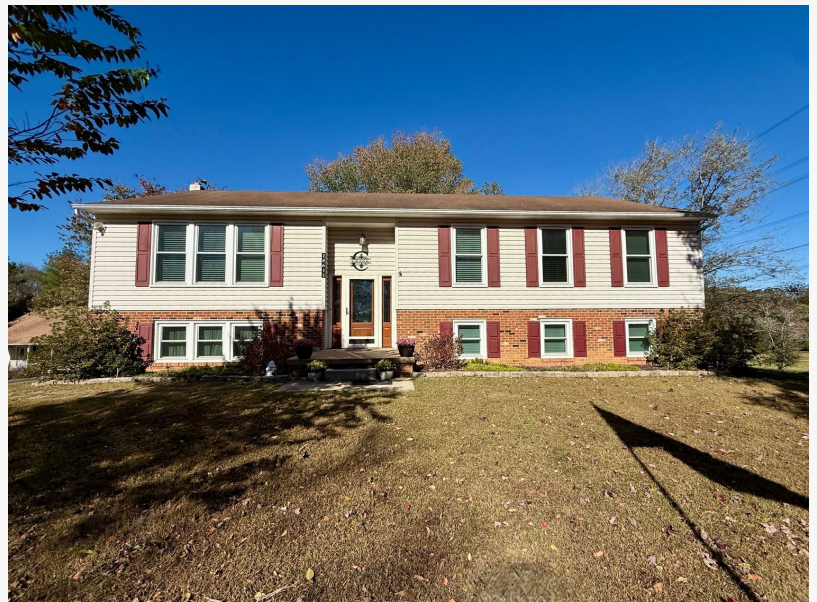
18611 Springs Rd., Jeffersonton, VA 22724 (Culpeper County)
