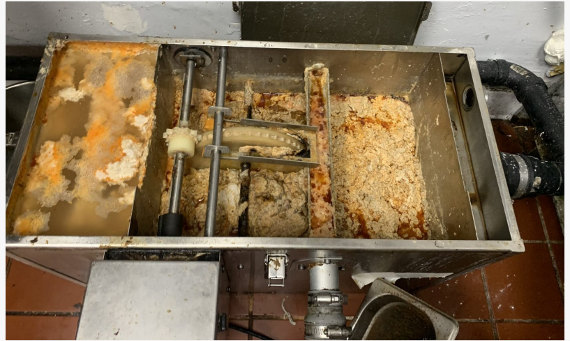
A full grease trap filled with fats, oils, and grease, highlighting the importance of regular grease trap cleaning and maintenance.
