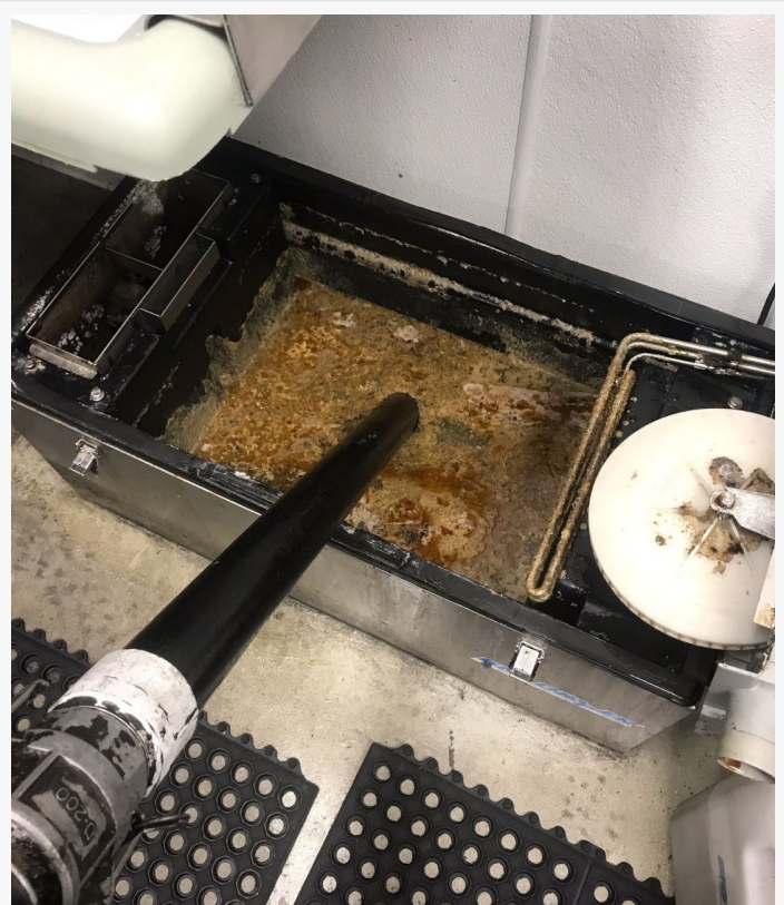
Technicians from Inland Empire Grease Company performing grease trap pumping to safely remove fats, oils, and grease from a commercial kitchen.
